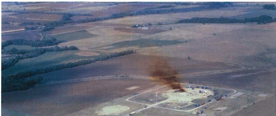
Figure 8: Aerial View of N_2O_4 Vapor Cloud Coming from Missile Silo 533-7
